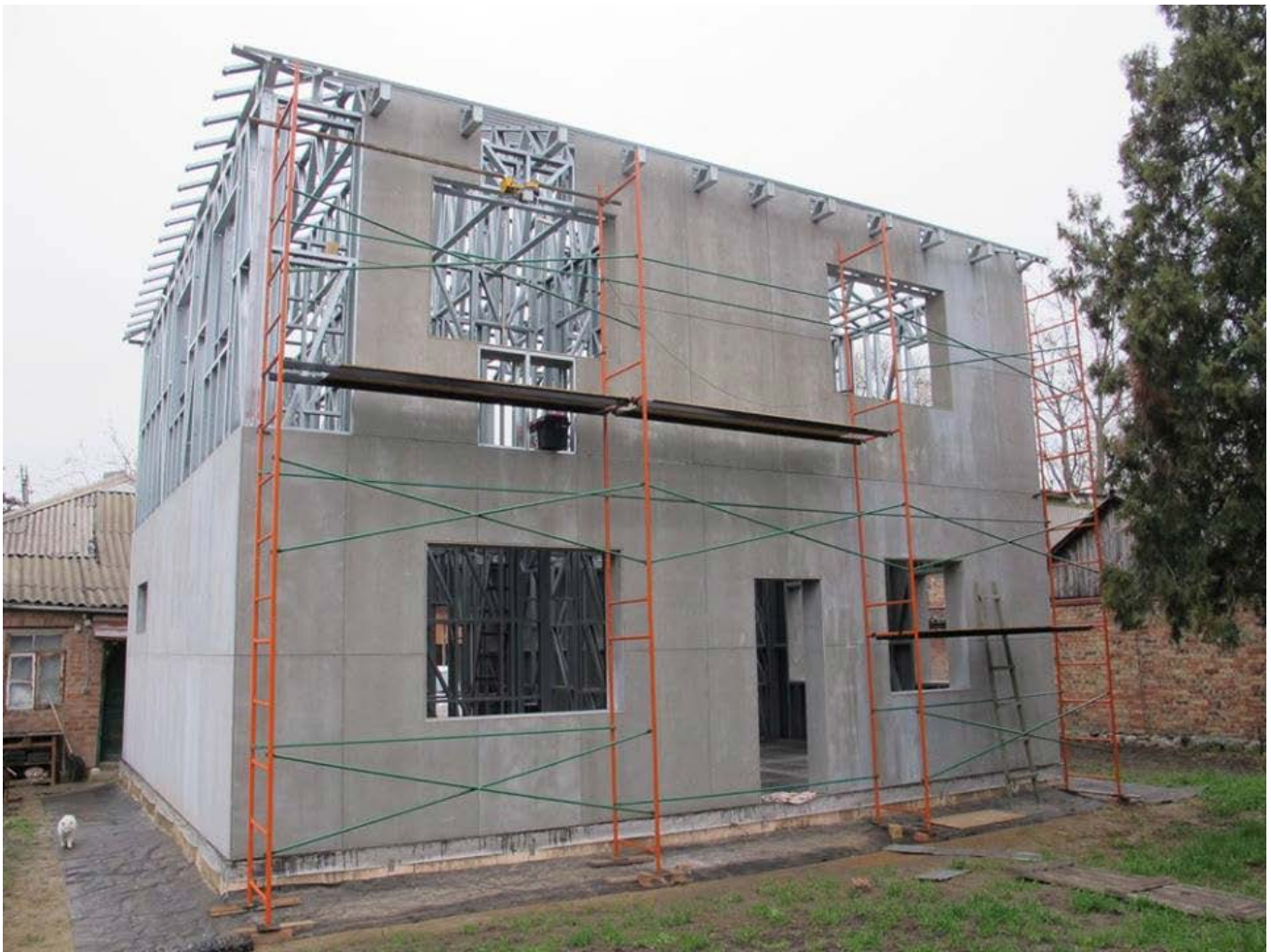
A Double Wall residential property with exterior facade being applied.
