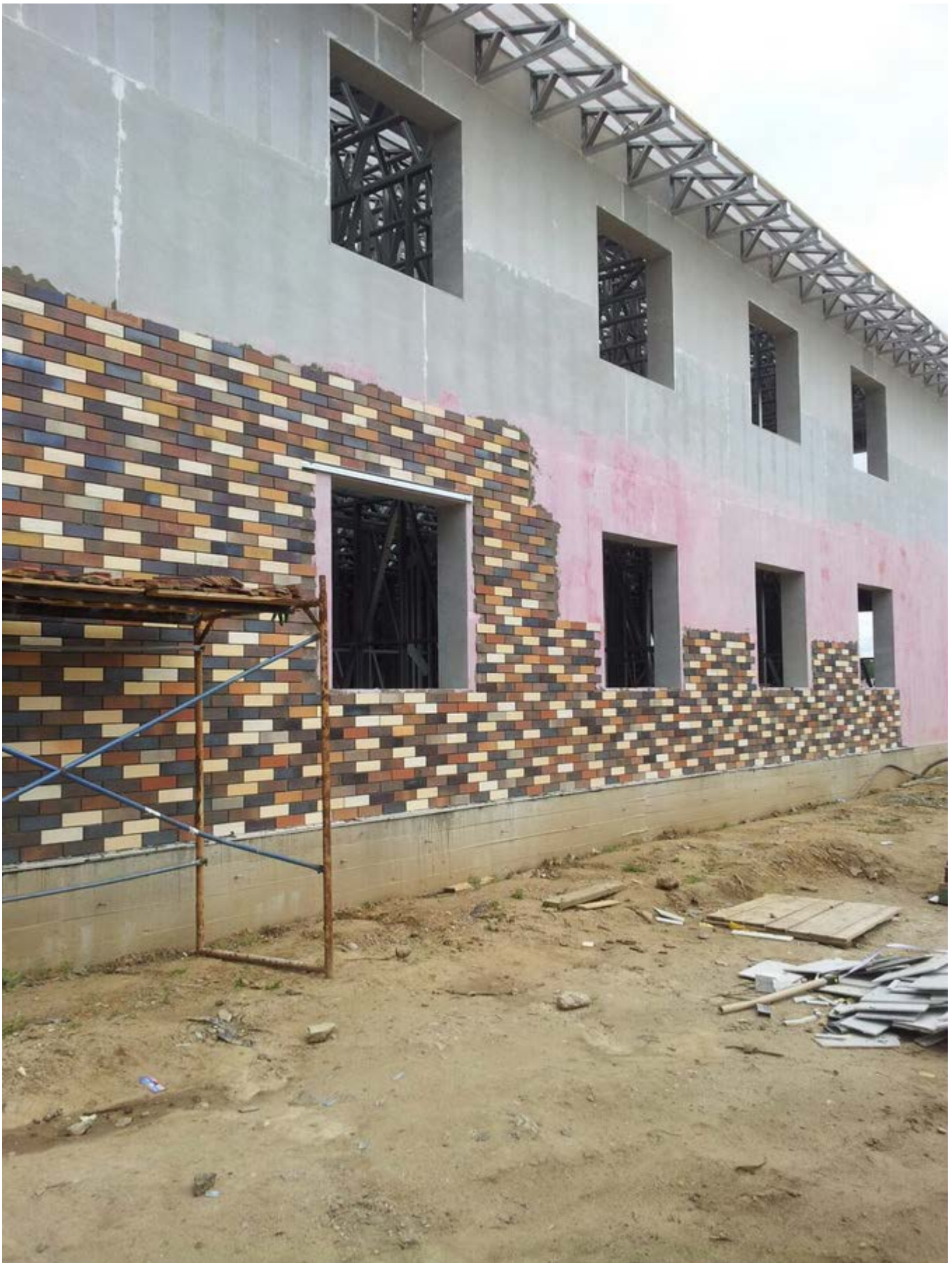
Standard finishes being applied to a Double Wall structure
