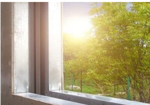
LGSF wall awaiting insulation and infill.
