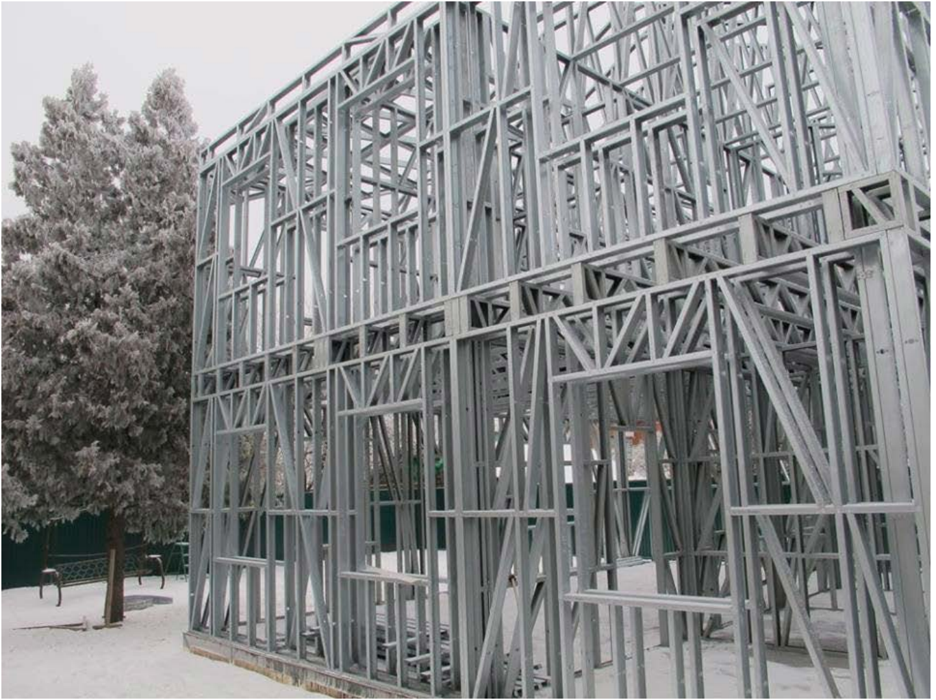
LGSF Double Wall residential building (note the snow/thermal conditions).
