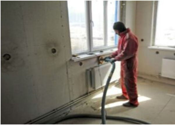
Insulation product being pumped into a Double Wall structure
